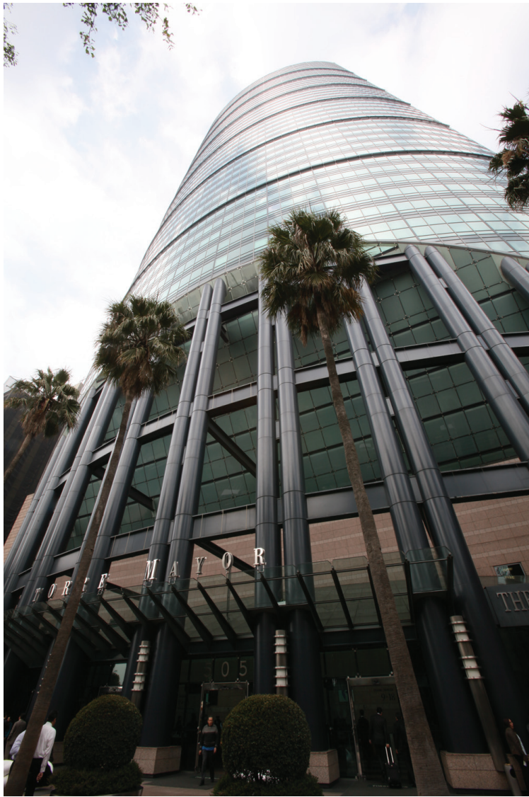
Torre Mayor in Mexico City is the tallest building in Mexico — and part-owned by Fibra UNO, the country's biggest REIT.
