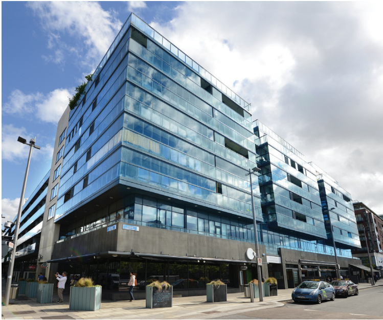
South Dock House in Dublin was acquired by Hibernia REIT in 2014 as part of a loan portfolio takeover from Ulster Bank.
