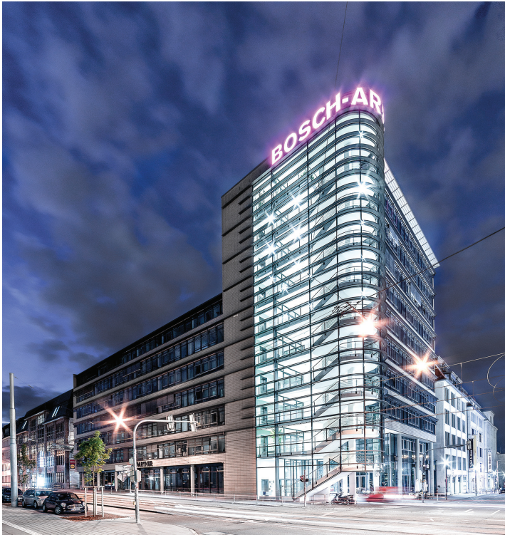
Schroder Real Estate has acquired the Bosch-Areal property in Stuttgart, Germany, for more than €100 million (US$113 million). The mixed-use property was acquired on behalf of a German client. Sascha Harms, head of real estate investment, Germany, with Schroders notes, “This asset is ... a relatively defensive component in our investment strategy and, given the strength of the Stuttgart leasing market, we are anticipating a highly-stable cashflow with upside potential from active asset management.”
